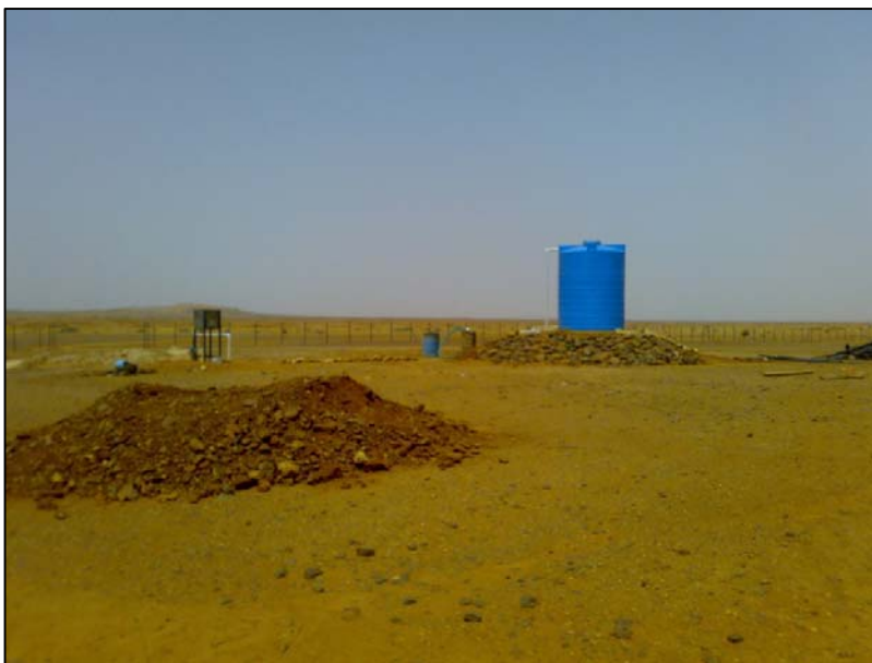
Plate 4.4: Observation Well constructed at one corner of the New Landfill site
